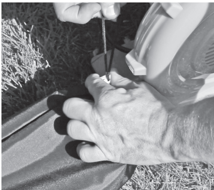
Tighten cinch cord around blower pipe
