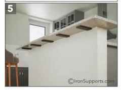
**3.** Place the bracket into the mounting channel and affix the bracket to the cap using ALL of the included #12 wood screws.
