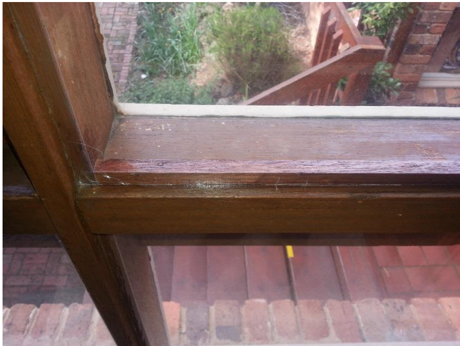
FIGURE 7: WINDOW FILM APPLIED TO WOODEN FRAME OF WINDOW
