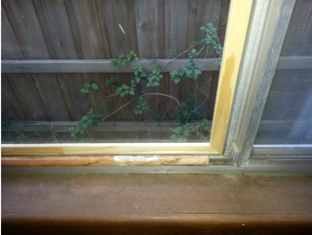
New internal wooden frame was installed at this property.
