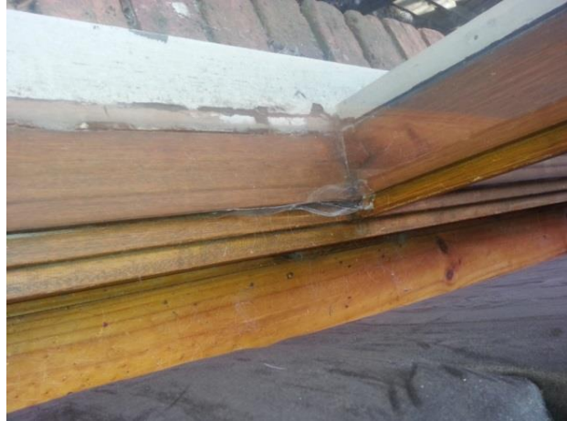
Rough unpainted timber
