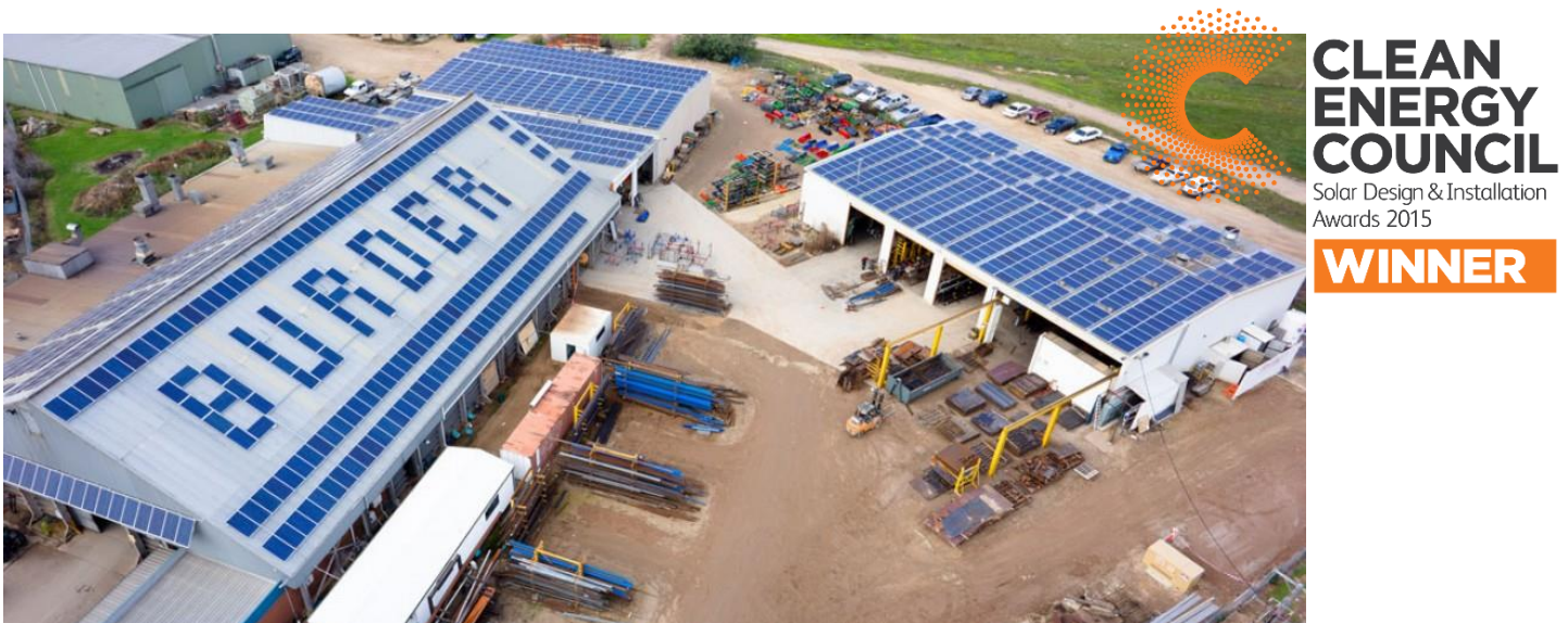
355 kW Solar PV System & Substation Upgrade (CEC WINNER – BEST COMMERCIAL INSTALLATION)
