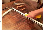
• Leave a tab of vinyl at the centre of each side. They can be handy for adjusting and remove the frame from the cavity later on. Trim off the excess vinyl with scissors.
