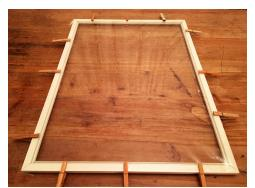
• Starting at a corner and working along the shortest edge first, push the spline into the gutter of the frame using the spline roller so that the vinyl is held firmly in place. Remove the pegs as you go. When you have made your way around the entire frame trim the spline off.
