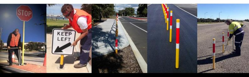
Use to secure any size or weight sign on a 60 OD post (from 150/350 mm depth); grab-rails (perfectly aligned) and traffic bollards (for use on highways) Any wall thickness, in speed zones from 10 kmph - 110 kmph. There are no limitations. Save time & money. NB: MRWA has approved the use of cheaper, more resilient CHS posts in all regions and Fibre reinforced posts in urban regions.
