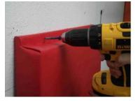
Fit your mats snugly beneath the pads when complete, if you need to make cuts to your mats, bury the cut edge underneath the wall pad, as the padding will overhang the mat edge by 1.5".
