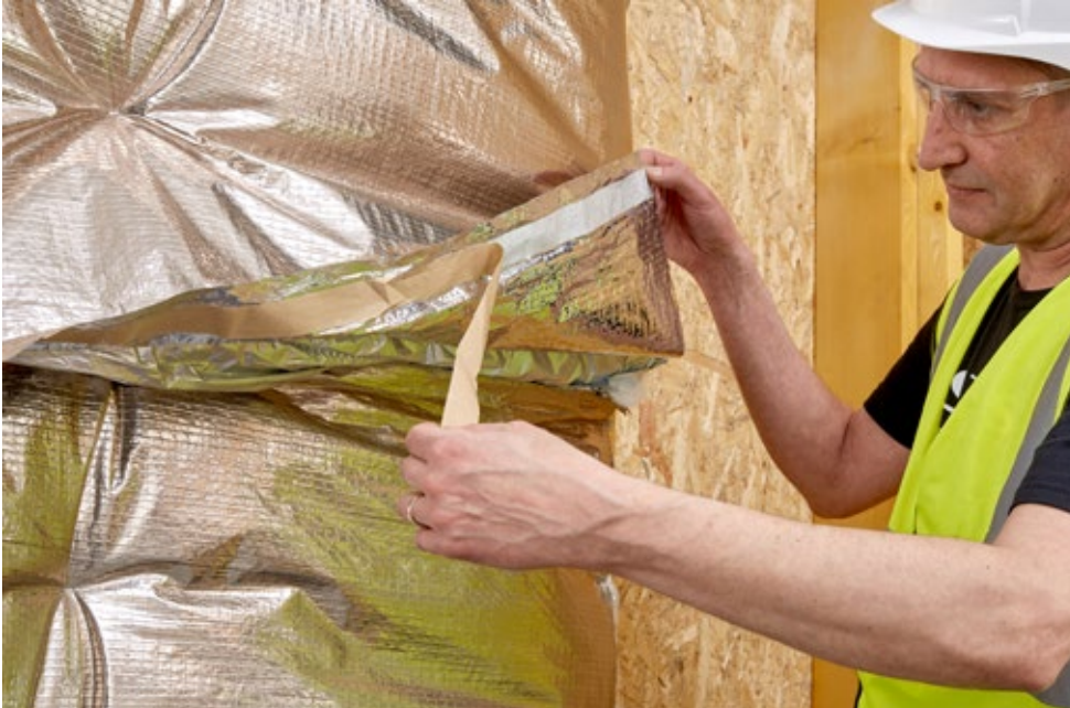
Overlap and seal with integral tape
