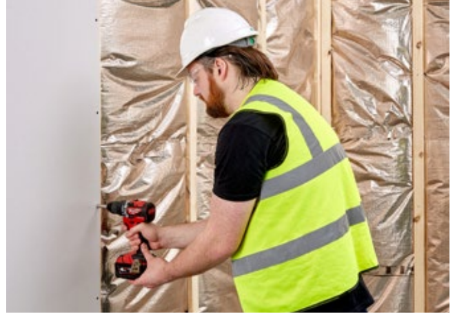
Fix plasterboard
