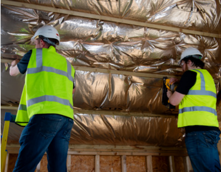
Prepare for plasterboard fixing
