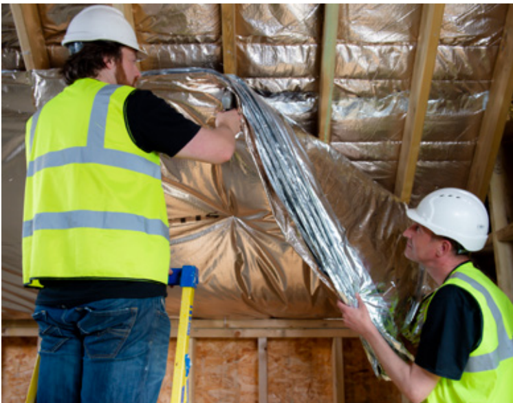
Install across rafters
