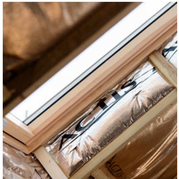
Perimeter edges: Stapled, taped, secured with batten
