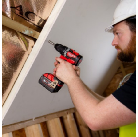
Fix plasterboard
