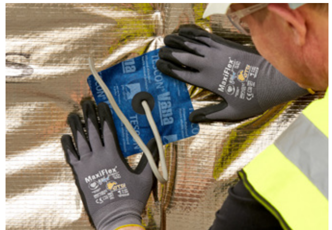
Fix grommet around electric wiring
