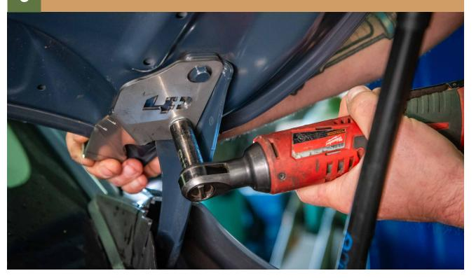
SPECIAL TIP: WHEN INSTALLING YOUR FOG LIGHTS ONTO YOUR NEW HOOD LIGHT BRACKETS. USE THE PROVIDED HOLES TO HELP SECURE THE CABLE
