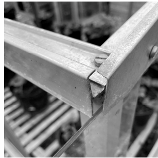
B Cold frame end glass fitting
