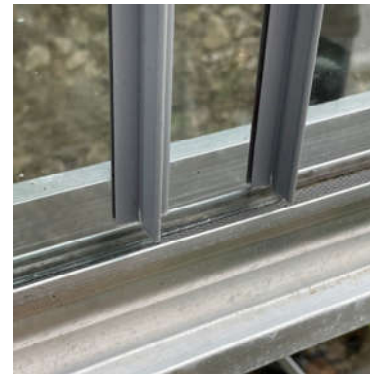
Glass in channel with two sheets overlapping
