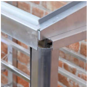
Corner trim in place
