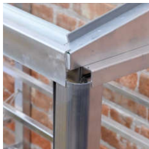
Corner trim in place
