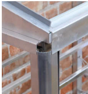
Corner trim in place
