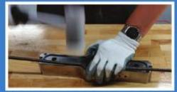
It is important to make sure the Nextflex heater is directly above the groove prior to striking. Form and install in 1 to 2 inch sections (25 to 50 mm).
