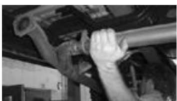
8. On 2016-19 trucks, remove the Hanger Bracket from the truck and Remount it to the forward position.
