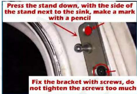
3. Remove the original struts and brackets. Mark the red dot as the picture shows and punch a hole by 9mm drill. Rivet gun pull rivet a nut.
