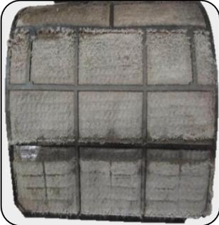
A photograph of a dirty U.I. filter. The white mesh filter is completely clogged with a thick, greyish-brown layer of dust and lint, making it almost unrecognizable. |
