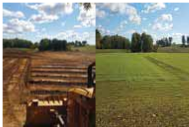
GROUND PREP ON NEW RESEARCH FARM
