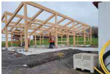
CONSTRUCTION OF NEW FULFILMENT CENTER
