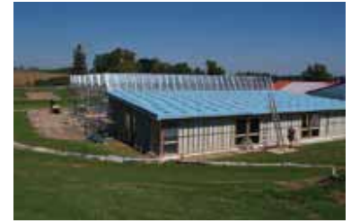
CONSTRUCTION NEW OFFICES AND GREEN
