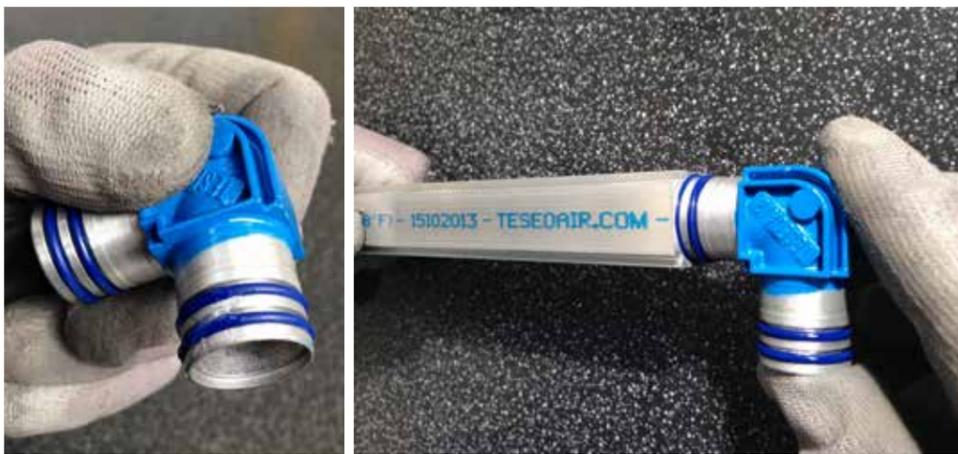
After the the two sections of pipe have been connected with the "L" joint, insert the provided "L" clamping bracket in the dovetails grooves and tighten the screws. The recommended tightening torque for M5 screws is between 10Nm and 13.5Nm. (Once the screw has come to a stop, make one more ¼ turn.)
