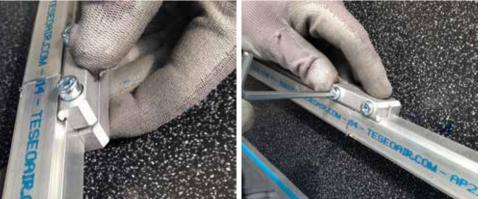
The screws should be tightened with the allen key. The recommended tightening torque for M5 screws is between 9 Nm and 11 Nm. Once the screw has come to a stop, make one more 1/4 turn. IN WARNING: After each joint is complete, check you have locked all the screws and not damaged the threads by over tightening.
