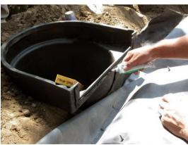
Easy liner attachment, clamps between spillway & housing (with sealant against the housing)
