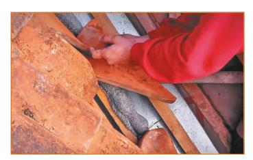
Place the pre-cut roof tile onto the Flexim with clean hands and press firmly into place. We recommend that the tile is mechanically secured.
