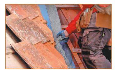
Press the Flexim onto a clean and dry substrate using the gloves provided. The width of the bonding area must be at least 5 cm.
