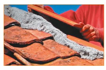
Place the ridge tile onto the Flexim with clean hands and press firmly into place.
