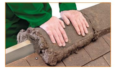
With clean hands, place the ridge tile onto the Flexim with and press firmly into place. Ensuring that Flexim is both inside and outside of the ridge-cap. Keep the joints as tight as possible
