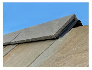
The first ridge should always be double fixed into position using 2 RidgeFix stainless steel screws with nitrile washers -
