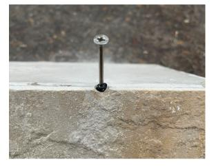
• Fix the second 60mm RidgeFix screw (supplied) through the ridge connector hole and into the batten.
