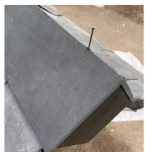
• Fix the second 60mm RidgeFix screw (supplied) through the ridge connector hole and into the batten.
