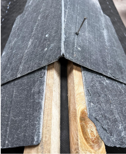
Installation with standard top battens
