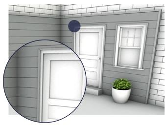
Installing the Corner Trims is the last phase of the project. Install the Composite Wall Cladding as above right up to any windows or doors.
