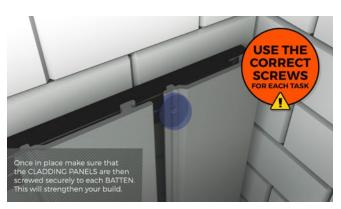
Ensure that the section between the Battens remains empty allowing air to flow beneath the Boards. Slot the second Board onto the first and repeat the fixing process ensuring that the second Board is fitted securely in place on each Batten. Repeat this process with each Board until you reach the required height.
