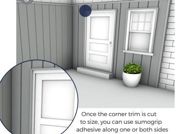
of the corner trim to attach to the edge of the cladding.
