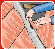
Adhering tiles or tile pieces to valleys
