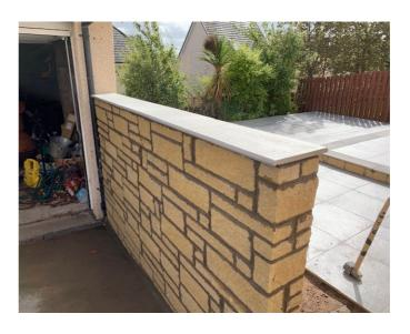
A bond bridge layer is required when laying in Mortar. We keep SBR bonding agent in stock for this purpose if required. The bond bridge should be created by mixing the SBR bonding agent into a slurry and painting it onto the back of each porcelain cope when laying.
