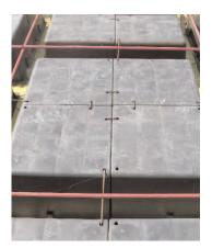
friendly"). The Wafflemat is created by connecting a series of Waffleboxes together, and evenly spacing them throughout the footprint area. A five inch post-tension reinforced concrete slab is then monolithically poured, the Waffleboxes allowing for any expansive soil movement. The pour also creates concrete beams running through the footprint and perimeter.
