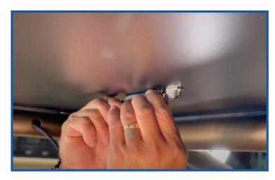
Make sure the plastic washer is on the bottom of the nut. Tighten with the wrench vertical as shown to prevent overtightening, which can strip or break the nut.
