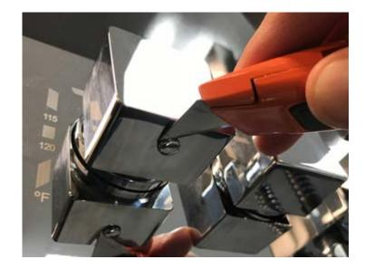
2. Using the alien key (included), unscrew set-screw and remove handles from the thermostatic valve and diverter.
