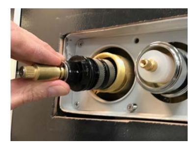
10. Place the new or cleaned out thermostatic cartridge back. Make sure to match the two white dots on the side. Place back the plastic safety ring, making sure that the two cutoffs are in vertical position.
