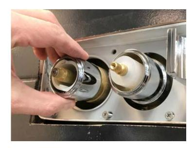
7. Pull out the safety plastic ring from the thermostatic valve.
