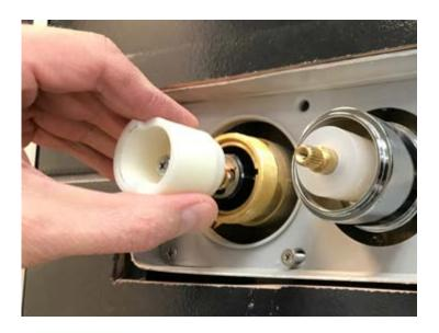
8. Using a small flathead screwdriver and hammer, carefully unscrew the ring nut from the thermostatic valve.
