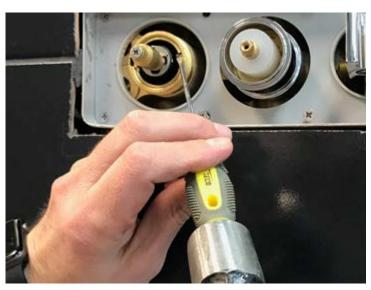
Pull out the thermostatic cartridge to replace it or clean it. Pliers might help if it's too tight. Rinse the system out before installing a new or cleaned cartridge.
