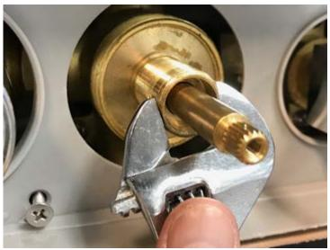
14. Pull out the diverter cartridge to replace it or clean it out.
