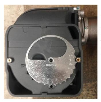
This is the first type. This type has to have the disc rotated to the C position to allow more airflow to be available with adjustment. If this is not done, you will NOT be able to attain the correct Co2 settings when commissioning the boiler.
