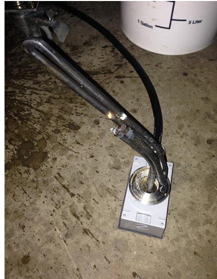
Figure 2: Complete heater failure
