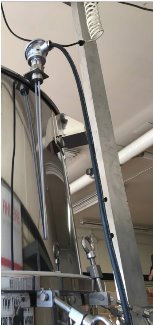
Figure 39: Water Level Sensor
