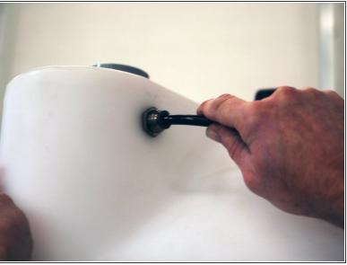
• Connect the "permeate" line to the bulkhead fitting in the water storage tank.
