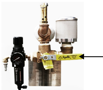
Ball valve in the open position
