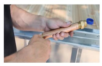
Wrap 3 layers of thread tape around the threads on both ends of the long pipe.
