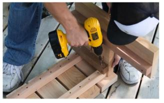
Ensure the stair support is flush at the back of the step and secure with  $2 - 2 \frac{1}{2}$ " (64mm) screws.
