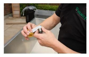
Wrap 3 layers of thread tape around the threads on both ends of the short pipe.
