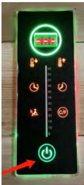
Sauna Control Panel is Illuminated
