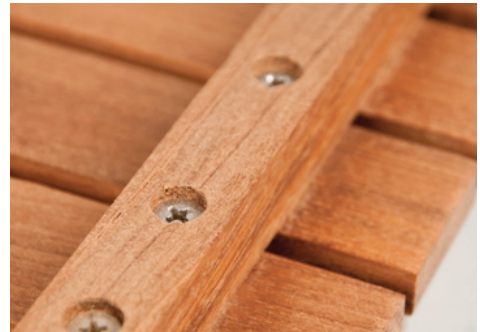
supports with countersunk screws
