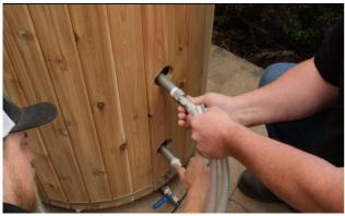
Connect the other ends of the chiller hoses to the tub. The hose from the outlet of the chiller will connect to the higher pipe of the tub and the hose from the inlet will connect to the lower pipe.
