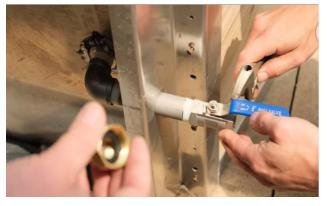
Using a pipe wrench or adjustable wrench, tighten the valve.
