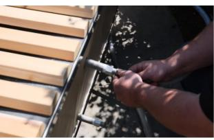
Connect the other ends of the chiller hoses to the tub.
