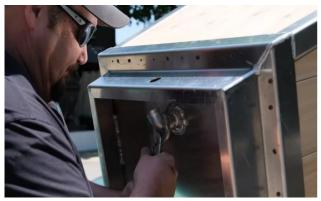
Screw the 90° elbow onto the short pipe.
