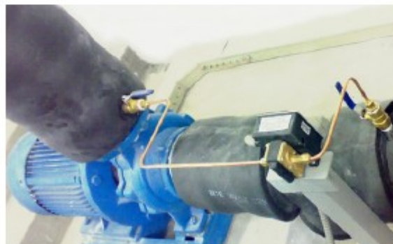
pump status detecting differential pressure flow switch installation
