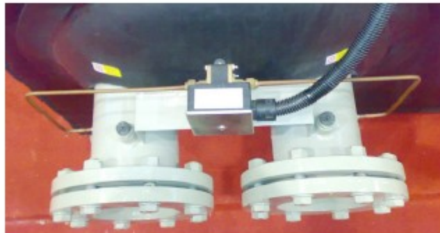
shell and tube type heat exchange differential pressure flow switch installation
