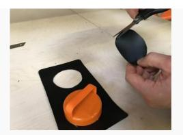
3. PUT PAINTER'S TAPE AROUND THE HOLE EQUAL TO THE DESIRED SIZE OF THE PATCH. USE THE CUT OUT PATCH AS A TEMPLATE.
