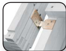
Installation on rafters
