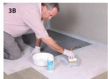
**3A.** Apply tape down the corner of the wall overlapping it where it meets on the tray. **3B.** Once taping is complete apply one coat of the TANKING<sup>™</sup> primer to the area that is to be tanked. This absorbs any dust and gives excellend ahesion for the tanking membrane
