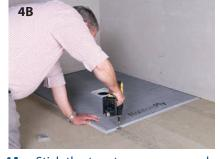
**4A.** Stick the tray to your prepared base using **MEGA** Strength Adhesive. **4B.** Secure the edges of the tray through the rebated section using the washers and screws provided. ONLY SCREW THROUGH THE REBATE SECTION. Run a thick bead of **MEGA** Strength Adhesive between the tray and walls.
