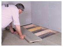
**1A.** Sweep the area clean, mark the position for your tray. **1B.** Cut free the floor boards and remove them. Fit extra timbers to support edge of existing floor if required.
