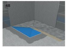
**4A.** When screed is set, remove 6mm rubber strip and fill gap with **MEGA** Power Sealant, plus gaps between the tray and walls. **4B.** The surface of the tray is primed ready to accept flexible tile adhesive and tiles.
