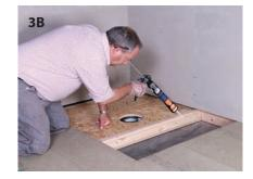
3A. Support the trap with timber to correct height, top of black seal should be flush with top of the joist.3B. Cut strips of OSB board to fit between joists and fix to battens
