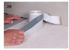
**2A.** Continue to fit your PrePrimed **No**More**Ply** across the rest of the floor until complete. **2B.** Apply the **MEGA** tape to all joints between tray and floor and between tray and wall. The split back makes it easy to apply and manipulate into corners.
