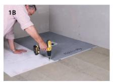
**1A.** Run a bead of **MEGA** Strength Adhesive along the rebated section on the two floor facing edges of the tray. **1B.** Lay your first sheet of Pre-Primed **No**More**Ply** board as per fitting instructions overlapping onto the rebate of the tray.
