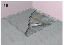
**1A.** Cut out concrete floor to the size of the tray, plus and entire 100mm in both directions about 40mm deep. Position trap and connect to waste. Fill around trap with weak sand and cement mix. **1B.** Lay a level bed of fast setting concrete, ensuring it is 32mm below existing floor level.
