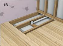
**1A.** Cut floor boards to the size of the tray and remove. **1B.** Position trap and support with timber to the correct height - top of rubber seal should be flush with top of joist.
