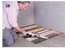
**2A.** Position the trap directly below the preformed drain opening and connect to the external waste. **2B.** Fix 2x1" PSE battens to each side of joists using **MEGA** Strength Adhesive and screws. Position the battens according to the thickness of your OSB board.
