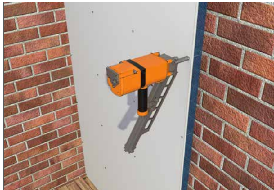
Fig. 4 Direct fixing Spacetherm Multi using nailgun
