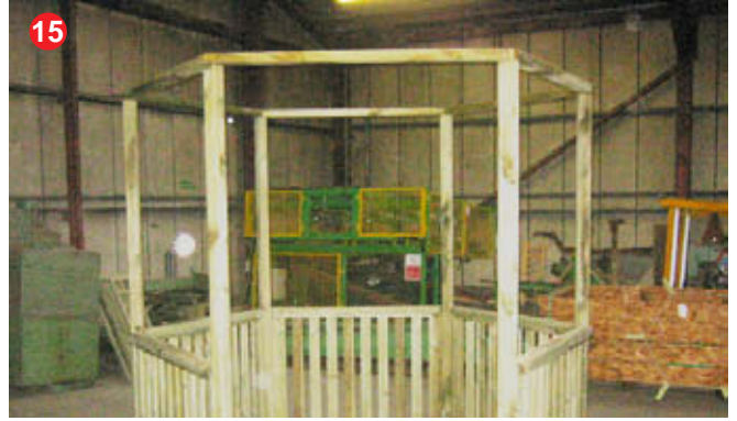
Upright top frames are positioned as shown.
