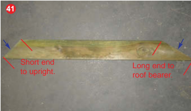
Drill a hole in each end of the 6 roof supports. Note the orientation.
