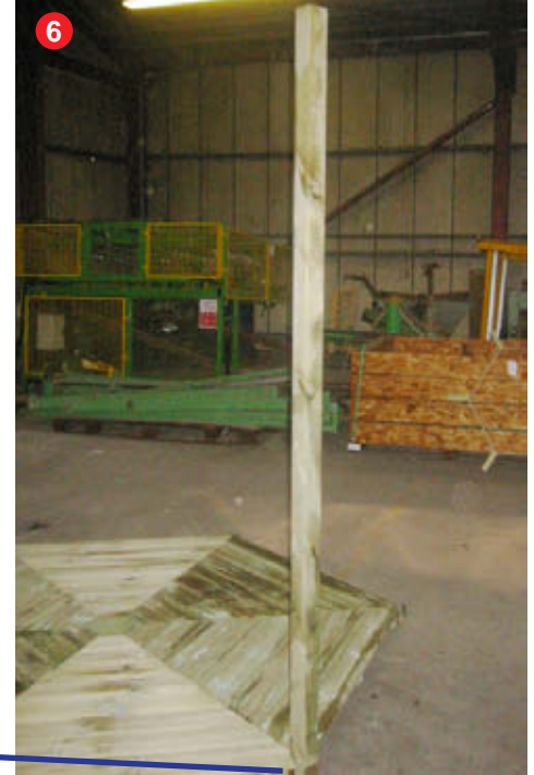
Uprights are located into the metal brackets.
