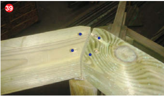
Secure small top frames to the top long roof bearers, using 4 x 70mm screws.
