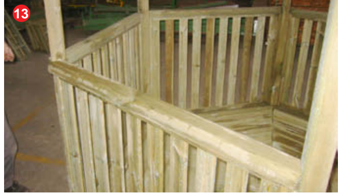
Position a handrail on top of each fence.
