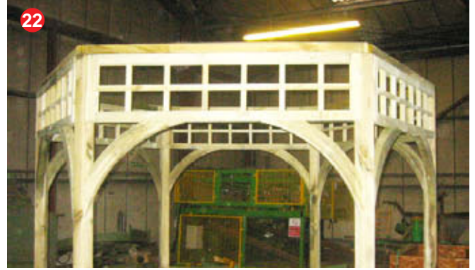
22 Attach arches using 2 x 40mm screws per arch.
